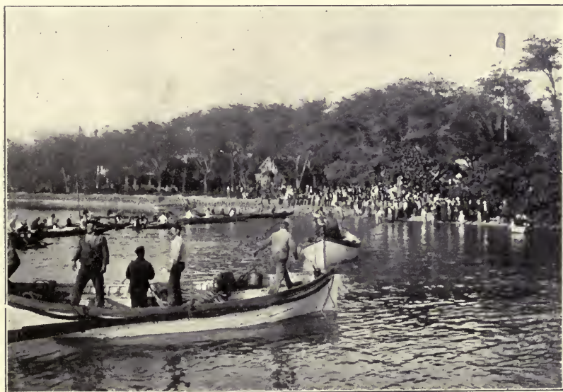
Hauling the rope ashore from cable-ship at Honolulu
